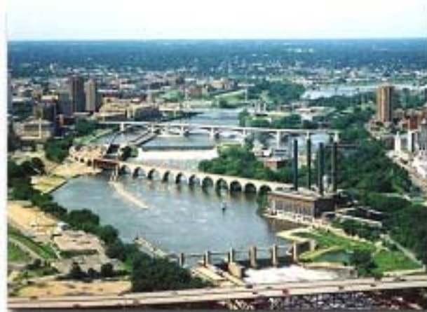
View of Upper St. Anthony Falls, Minneapolis, MN (photo courtesy of US Army Corp of Engineers)
