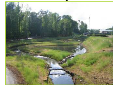
Completed floodplain wetland showing off-channel storage of stream flow.
